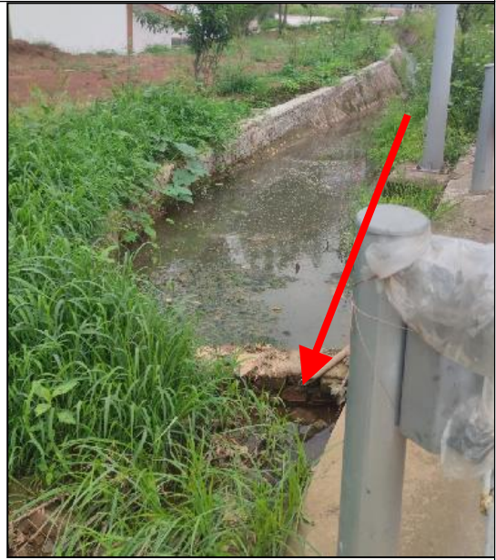
PDK0+490.471~PDK0+515.471 段堵塞圆管涵
